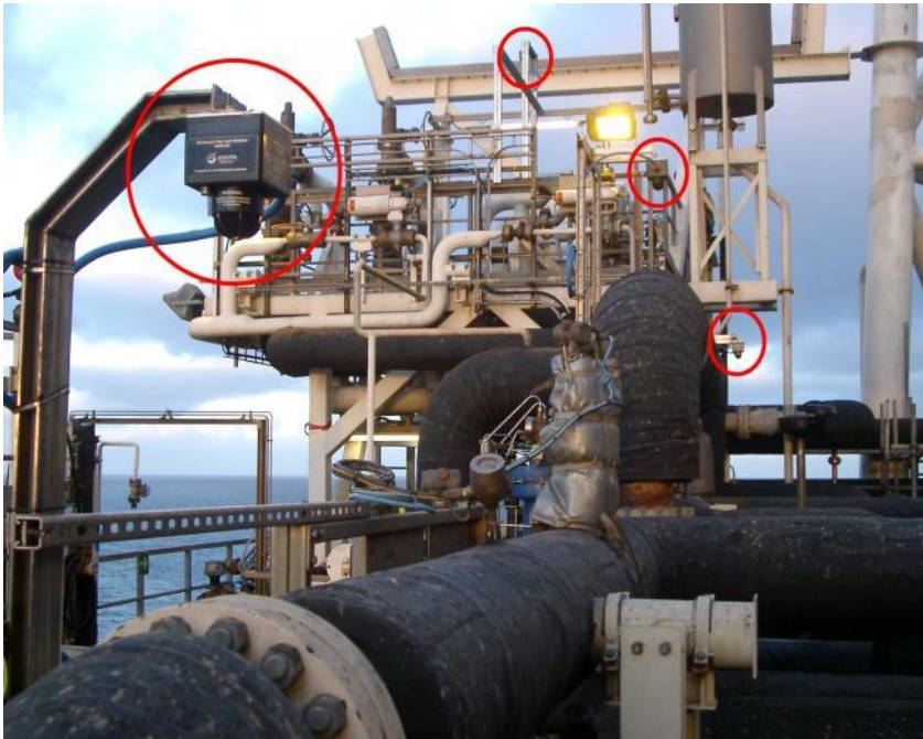
7 out of 9 Ultrasonic detectors installed on a Hess weather deck in the North Sea.
